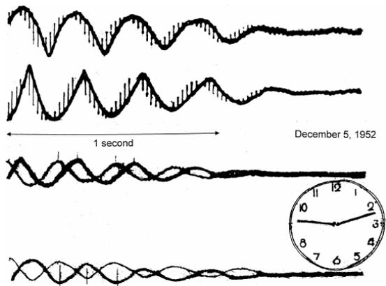
Figure 5 A typical wind record photographed onto moving 70mm wide recording paper in 1952.
